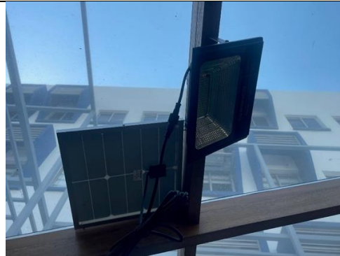
Solar panels installation an example of renewable energy
